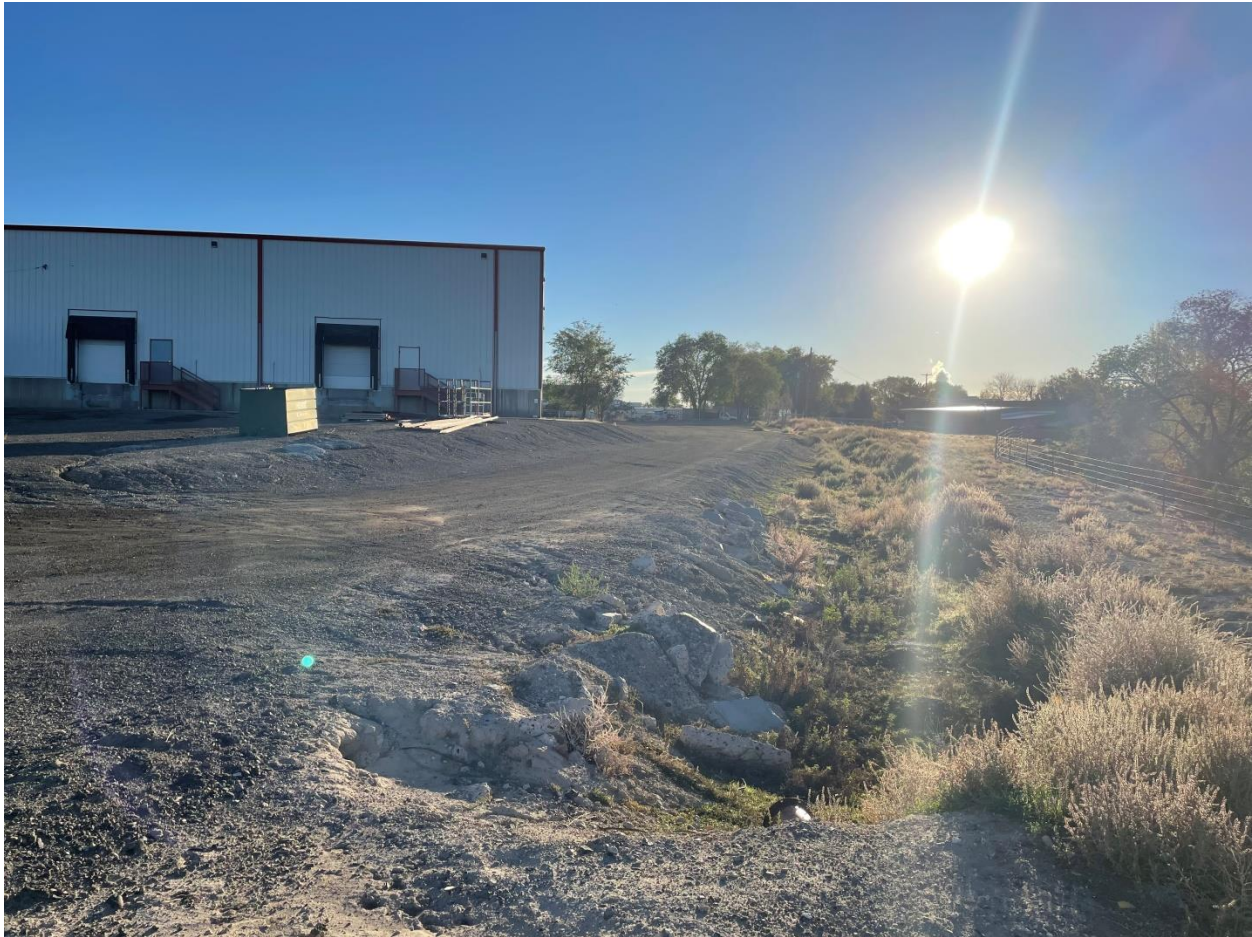
West Side of the Existing Building Looking East
