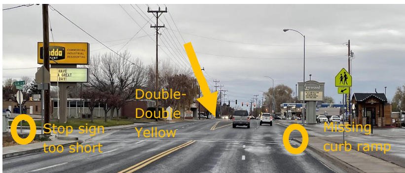
FIGURE 17: FILER AVENUE AND ELM STREET N ISSUES
