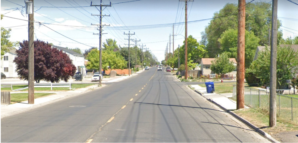
FIGURE 7: UTILITY POLES IN SIDEWALKS
