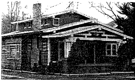
Dormers should be placed in from the eave line of the house, as these original dormers illustrate.
