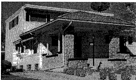
A second story addition that follows the pitch and roofline of the main part of the house, and is set back from the plane of the front wall, will go a long way from detracting from the historic appearance of a house (above). Additions like this are incompatible with the massing and form of the original house, and should not be constructed (below).
