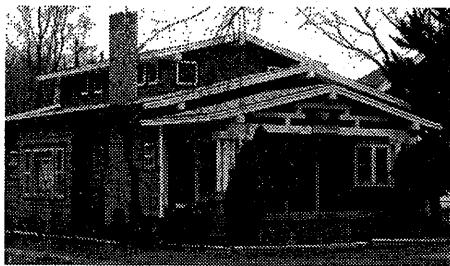
Dormers should be placed in from the eave line of the house, as these original dormers illustrate.
