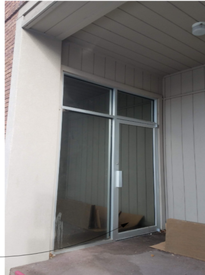
EXISTING ALUMINUM STOREFRONT DOOR IN ALCOVE ON GOODING ST. N.
