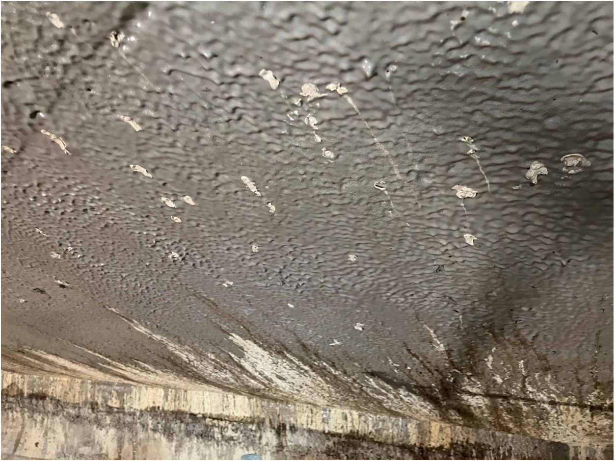
Photo 8: White pinhole repair material on digester cover interior
