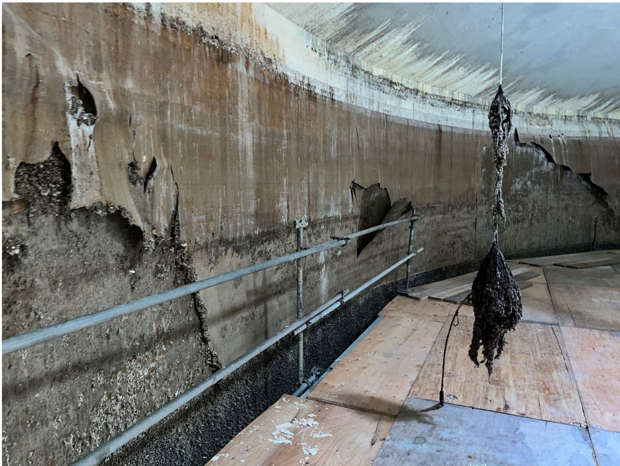
Photo 1: Overall view of digester skirt interior (prior to existing coating removal project)
