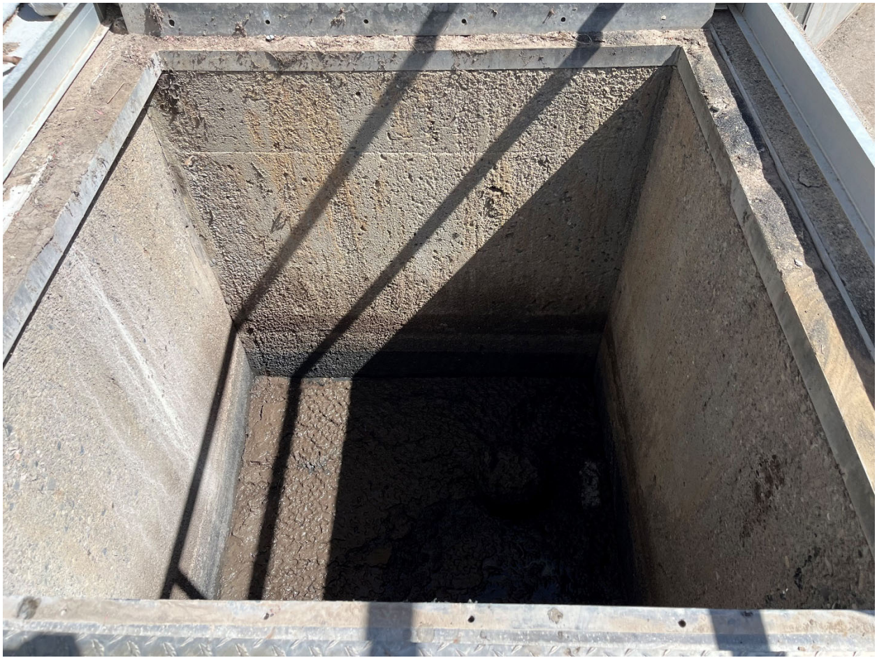
Photo 21: Overall view of digester overflow box
