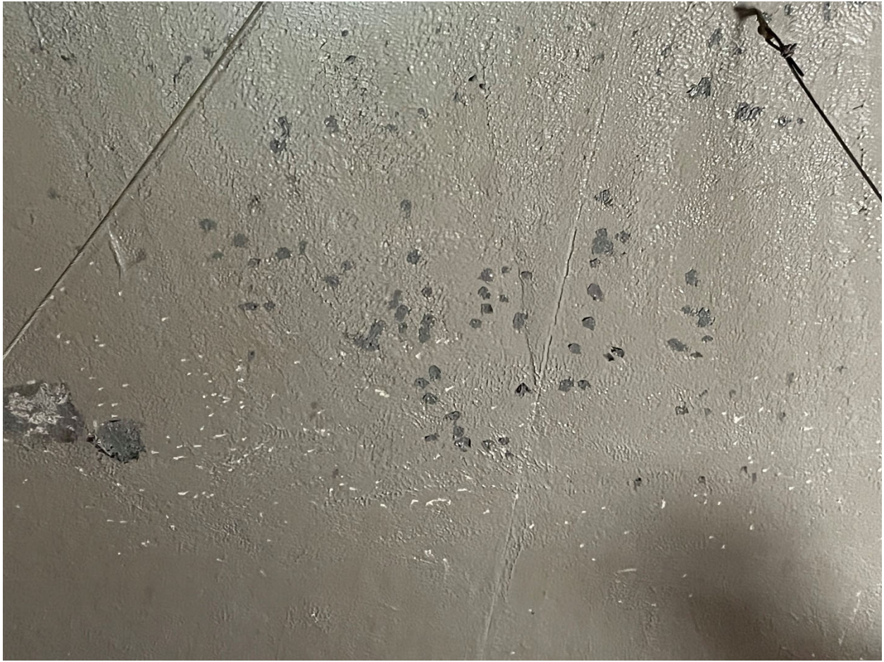
Photo 7: Grey pinhole repair material on digester cover interior
