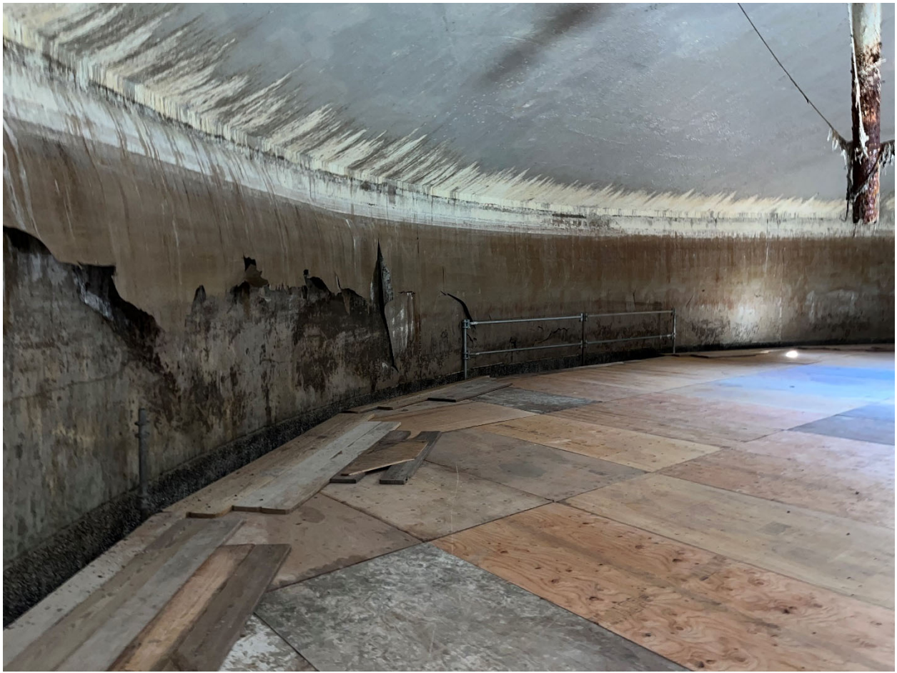
Photo 2: Overall view of digester skirt interior (prior to existing coating removal project)
