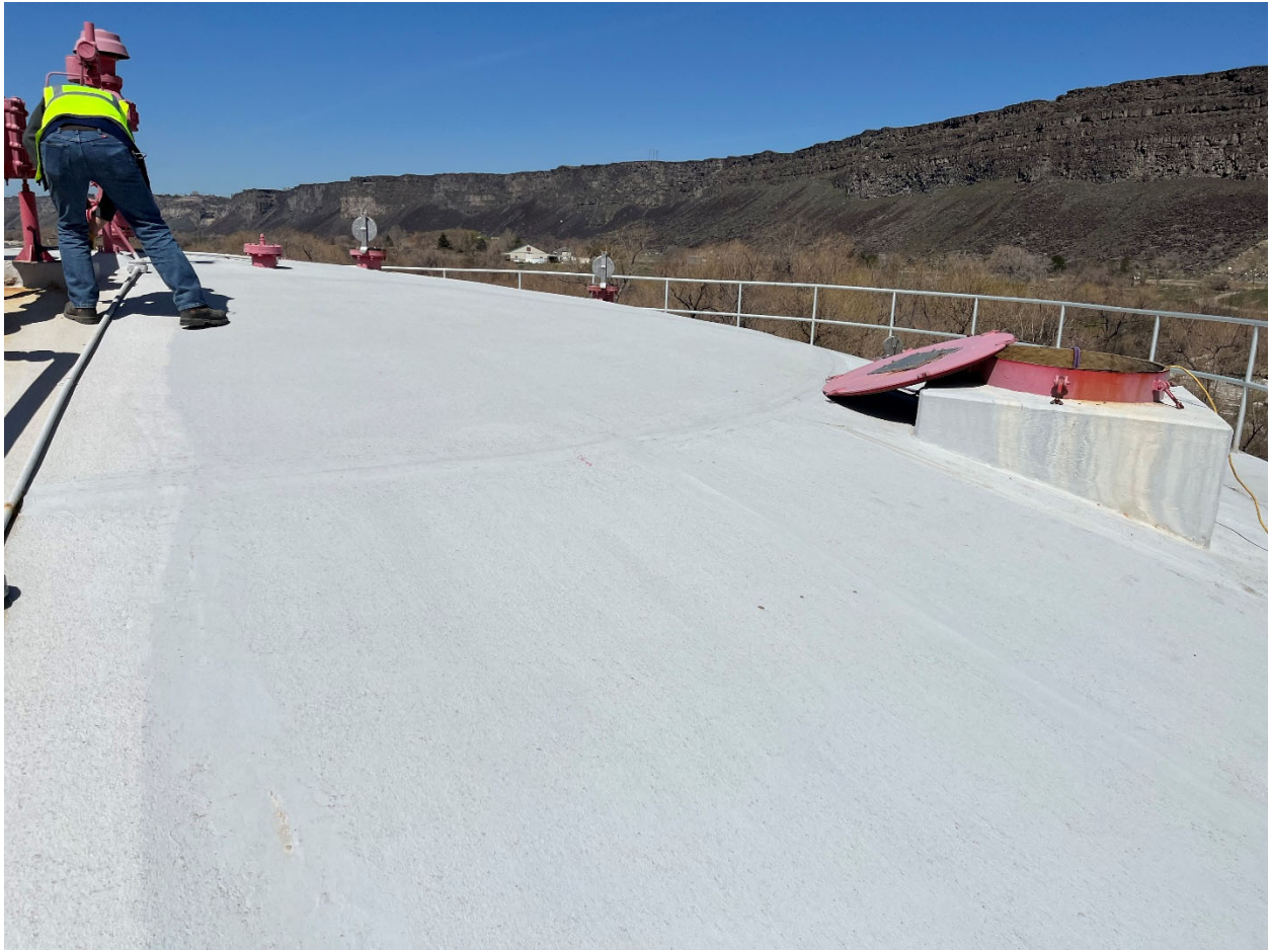
Photo 13: Overall view of digester cover exterior
