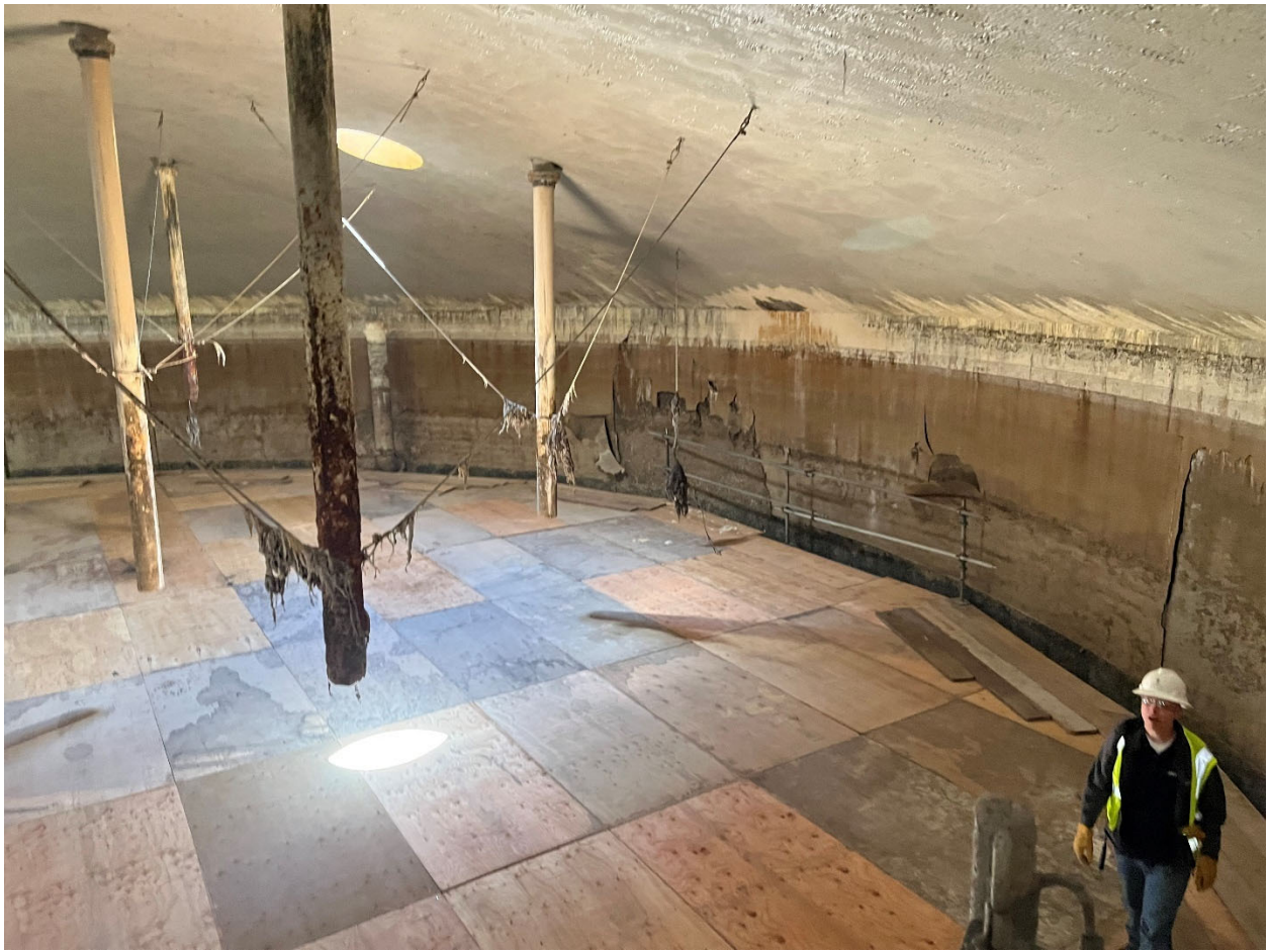
Photo 6: Overall view of digester cover interior
