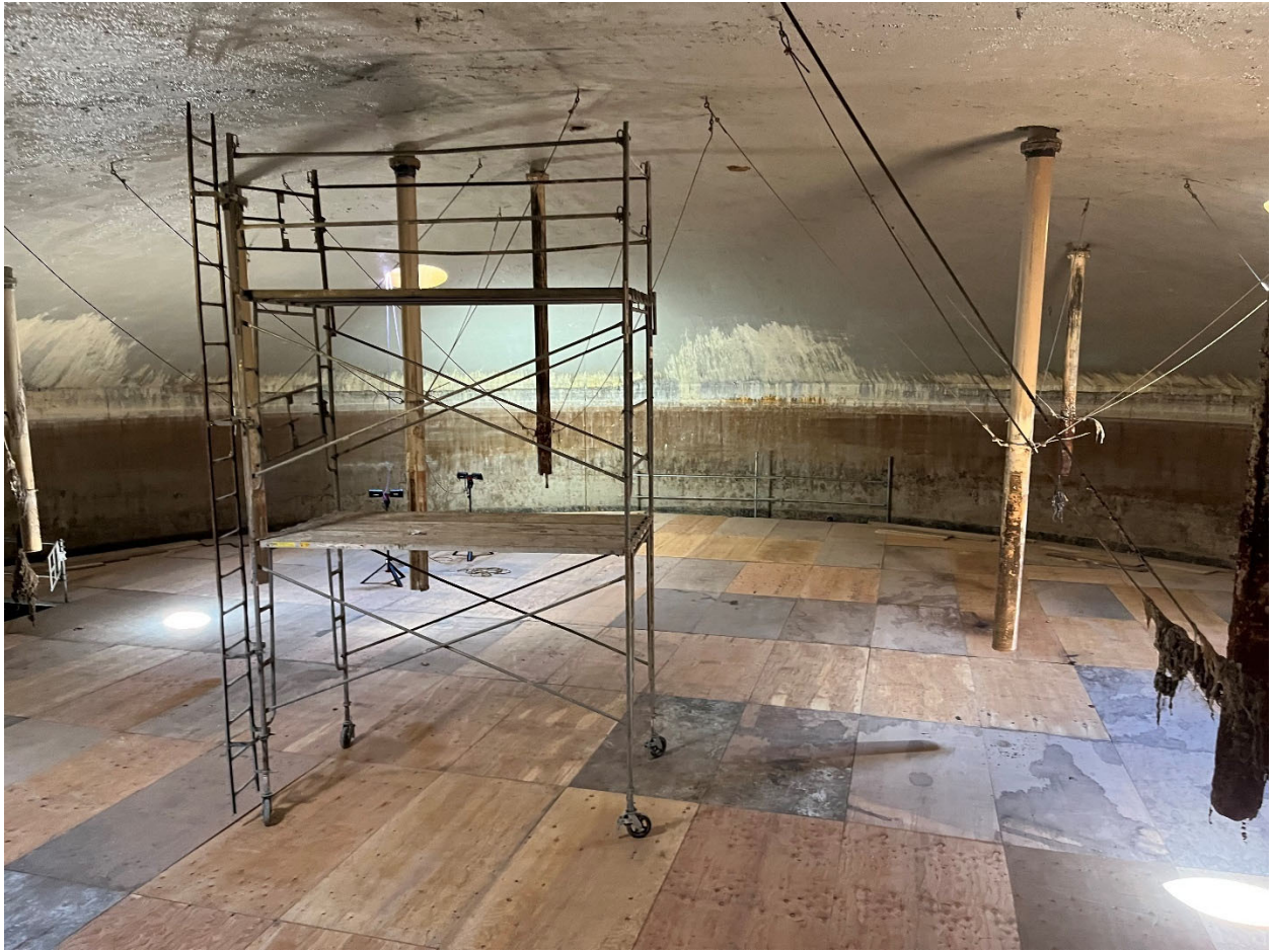
Photo 5: Overall view of digester cover interior
