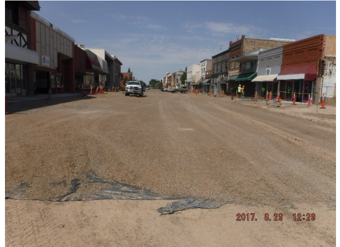
Block 3 – Shoshone to Hansen, base material placed and preparing for asphalt, 29AUG2017
