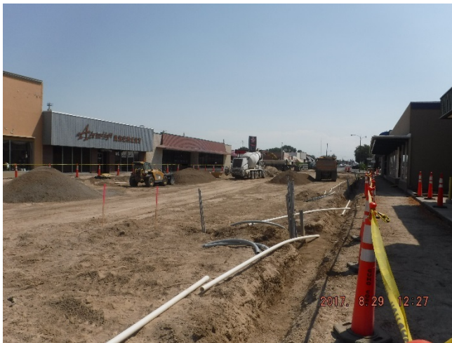
Block 4 – Hansen to Idaho, installing underground utilities, 29AUG2017
