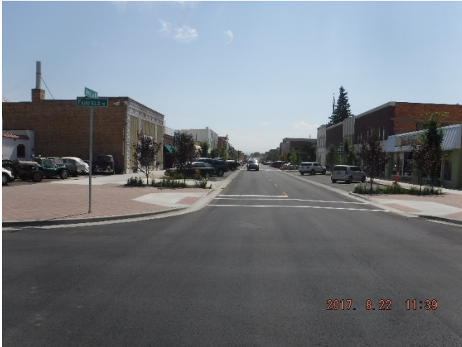
Block 2 – Gooding to Fairfield, block is open to traffic, installation of lights remains 22AUG2017
