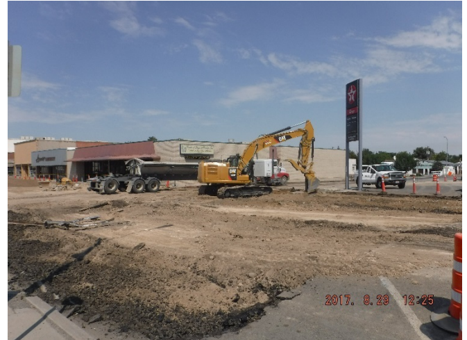
Block 5 – Idaho to Jerome, asphalt pavement demolition, 29AUG2017
