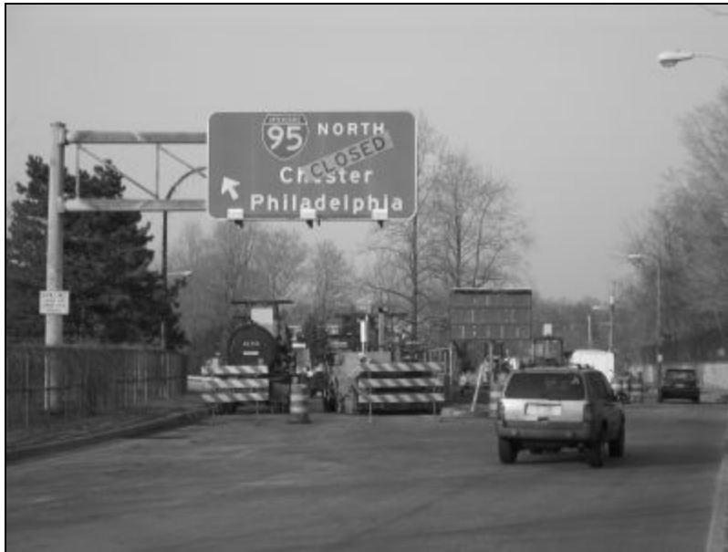
Figure 15 - I-95 North closed for construction
