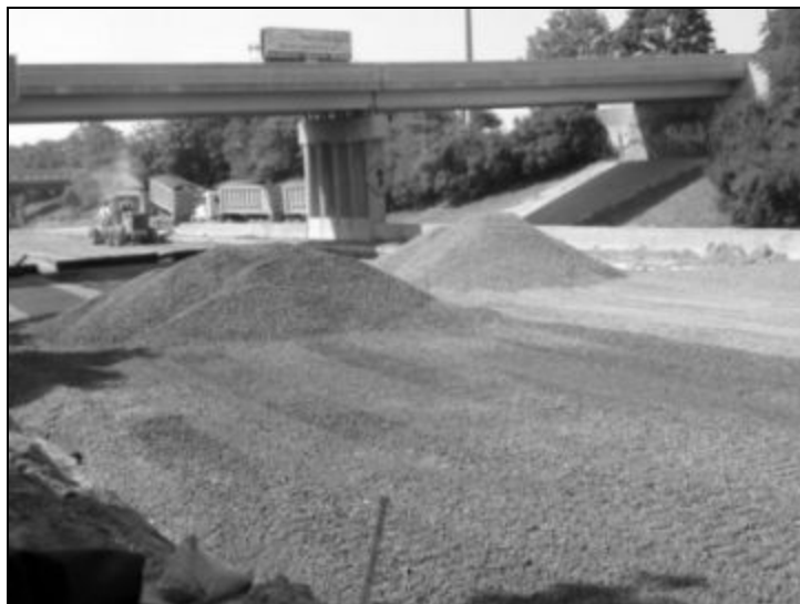
Figure 1 - Full closure increases available workspace for equipment and material
