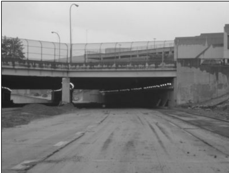
Figure 8 - The M-10 (Lodge Freeway) under full closure
