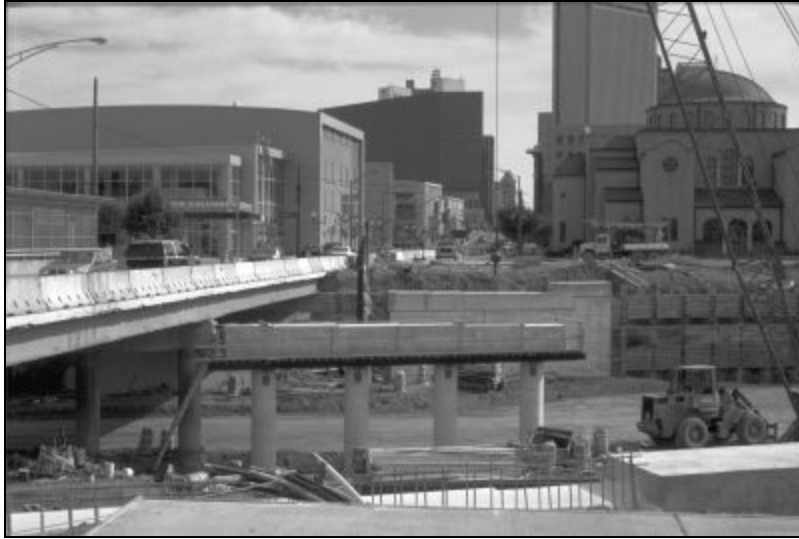
Figure 11 - Traffic crossing over the I-670 under full closure
