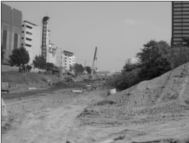
Figure 9 - Work being performed on the M-10 (Lodge Freeway) under full closure
