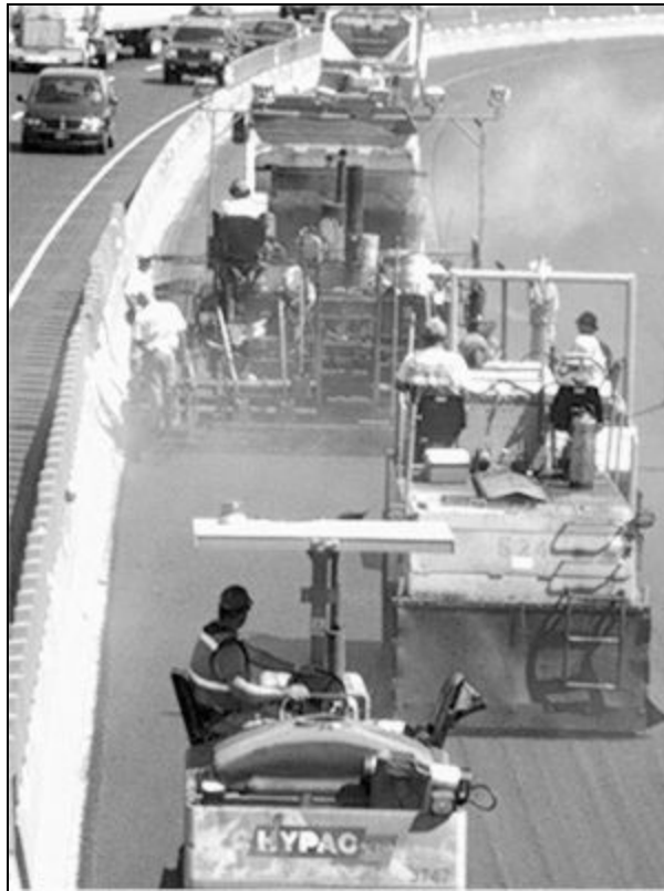
Figure 4 - Approximately 40,000 tons of asphalt were delivered in less than 100 hours
