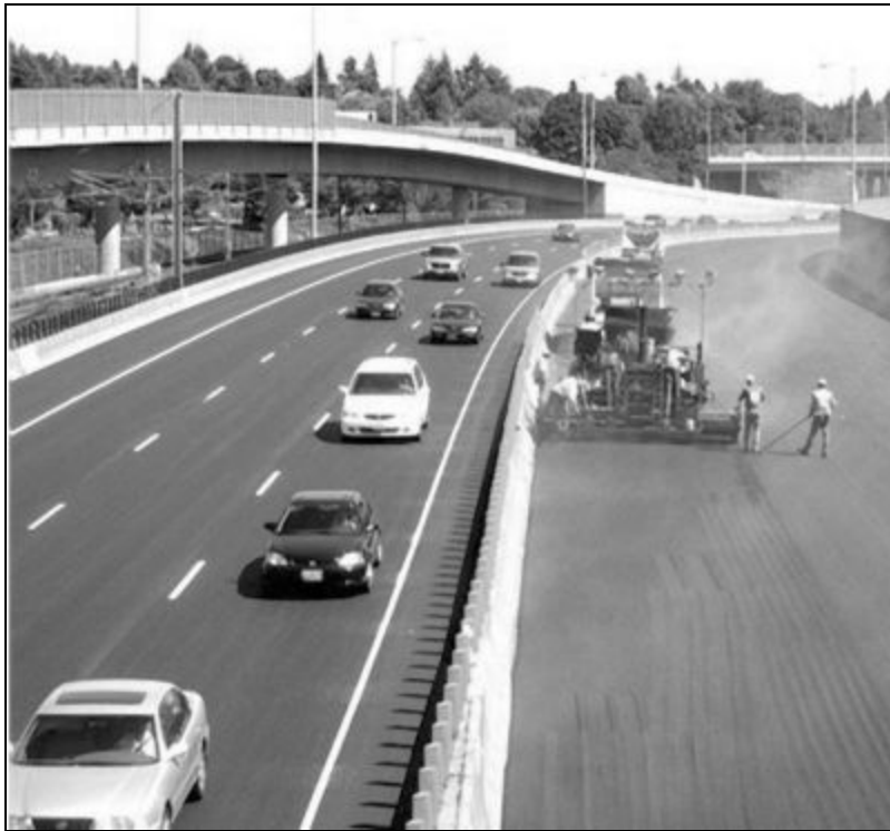
Figure 3 - Crews work without interruption on the I-84 (Banfield Freeway)
