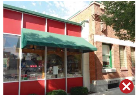
Inappropriate material selection.
