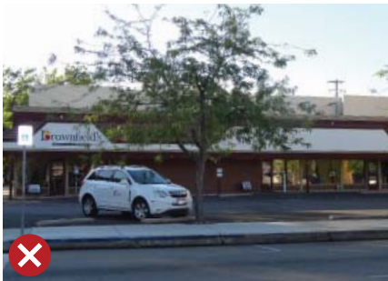
Inappropriate parking lot on street side.
