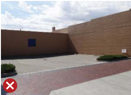
Inappropriate lack of screening.
