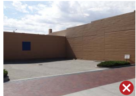
Inappropriate screening of off-street parking.
