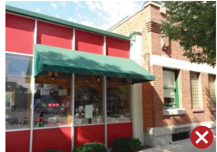
Inappropriate material selection.
