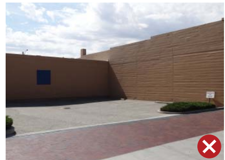
Inappropriate screening of off-street parking.
