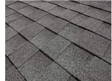
Existing Asphalt Roofing
