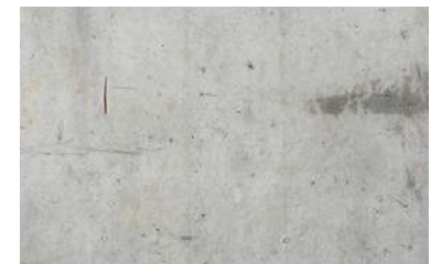
Existing Concrete Stem Wall Base
