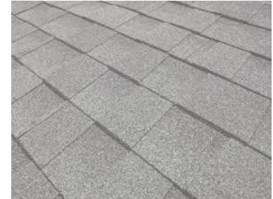
Existing Asphalt Roofing
