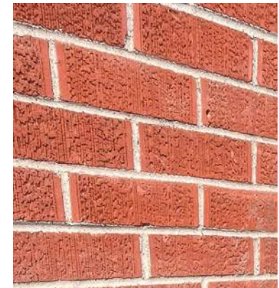
Existing Brick Wall
