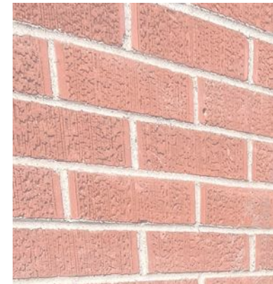
Existing Brick Wall
