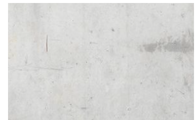
Existing Concrete Stem Wall Base
