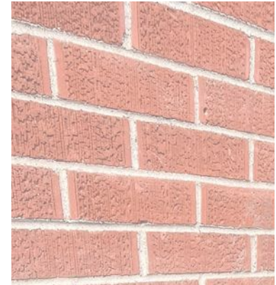
Existing Brick Wall
