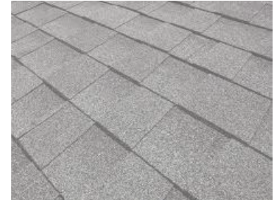
Existing Asphalt Roofing
