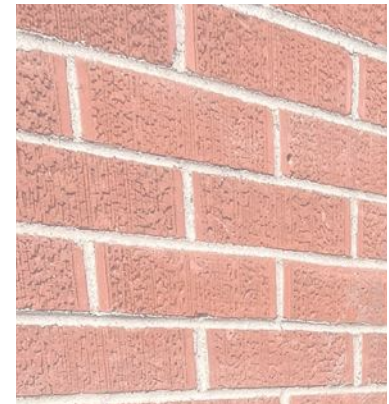
Existing Brick Wall
