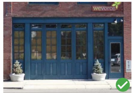
Appropriate historic bay in-fill.
