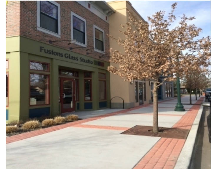
Eagle: Right-of-Way Improvements
