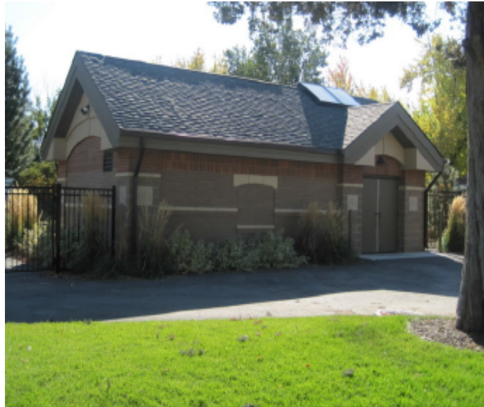
Garden City: City Well Rehab
