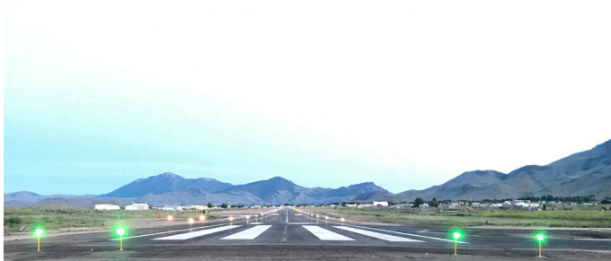
Challis Airport | Runway Reconstruction & Lighting
