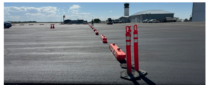
Magic Valley Regional Airport | Apron Expansion
