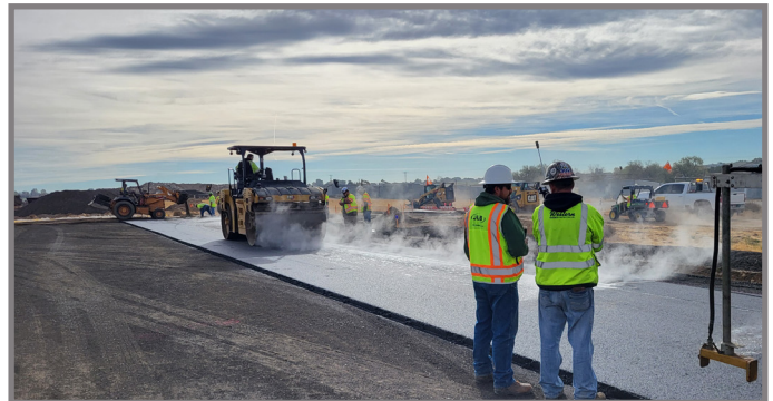
Buhl Municipal Airport | Reconstruct Runway
