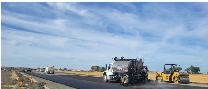
Buhl Municipal Airport | Runway Reconstruction & Lighting
