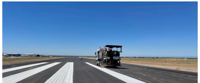
Jerome County Airport | Runway Rehabilitation & Lighting
