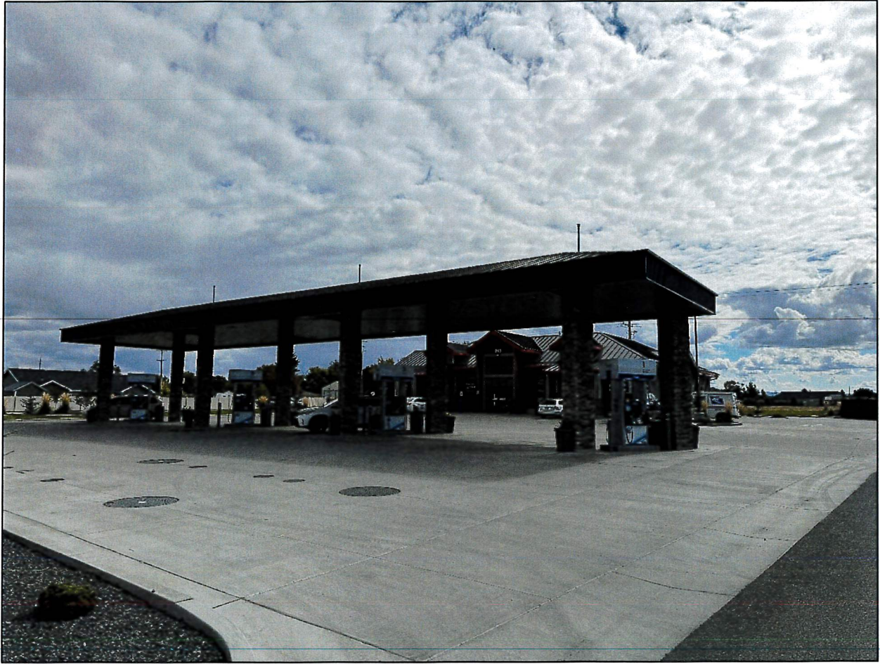
Figure 4 - Sample Elevation of similar style service station Example facility is Base Camp Twin Falls located at 915 Magic Rd, Twin Falls, ID 83301
