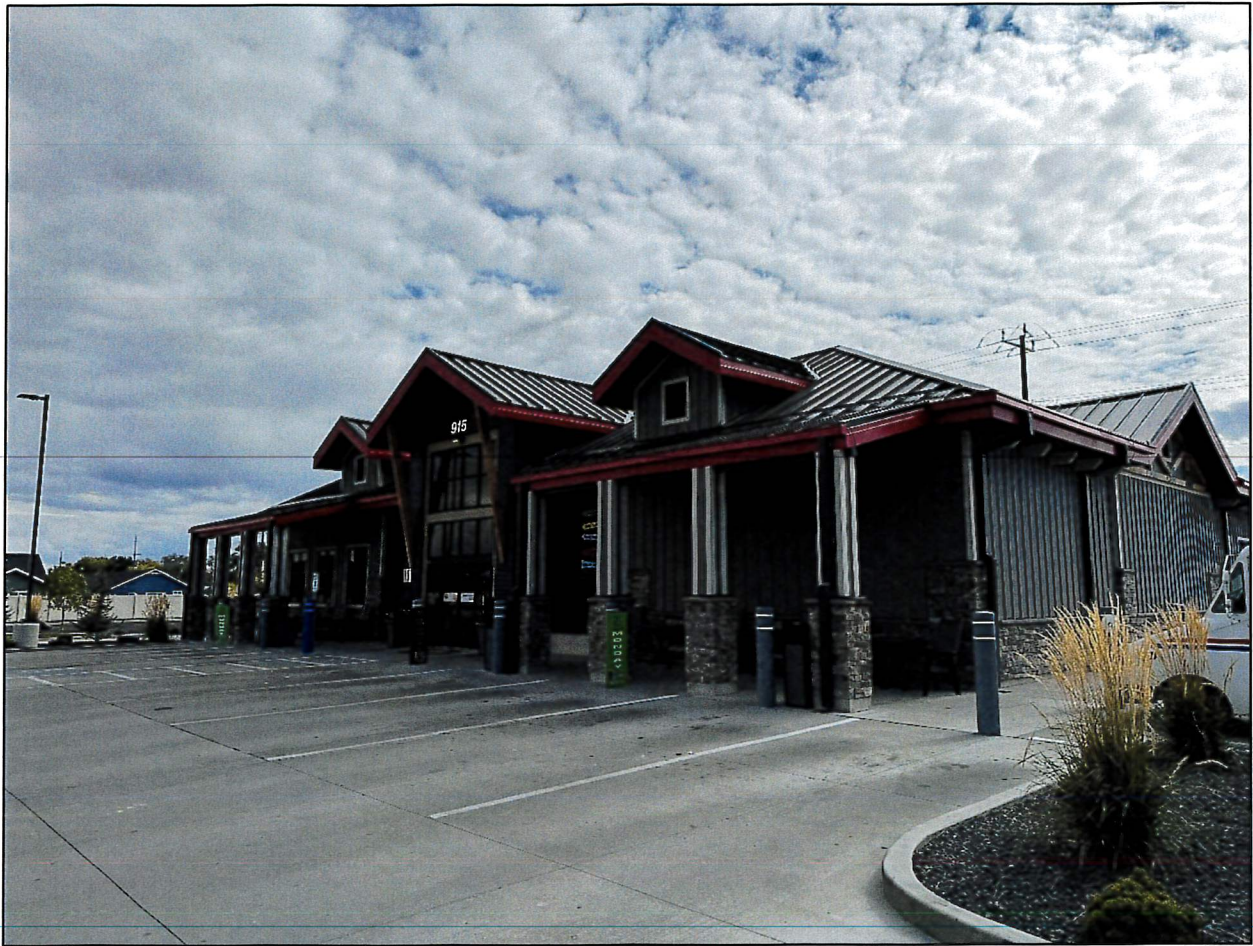
Figure 3 – Sample Elevation of similar style service station Example facility is Base Camp Twin Falls located at 915 Magic Rd, Twin Falls, ID 83301
