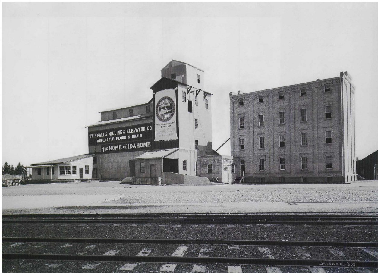
Twin Falls Milling and Elevator Company Warehouse Building is gone.
