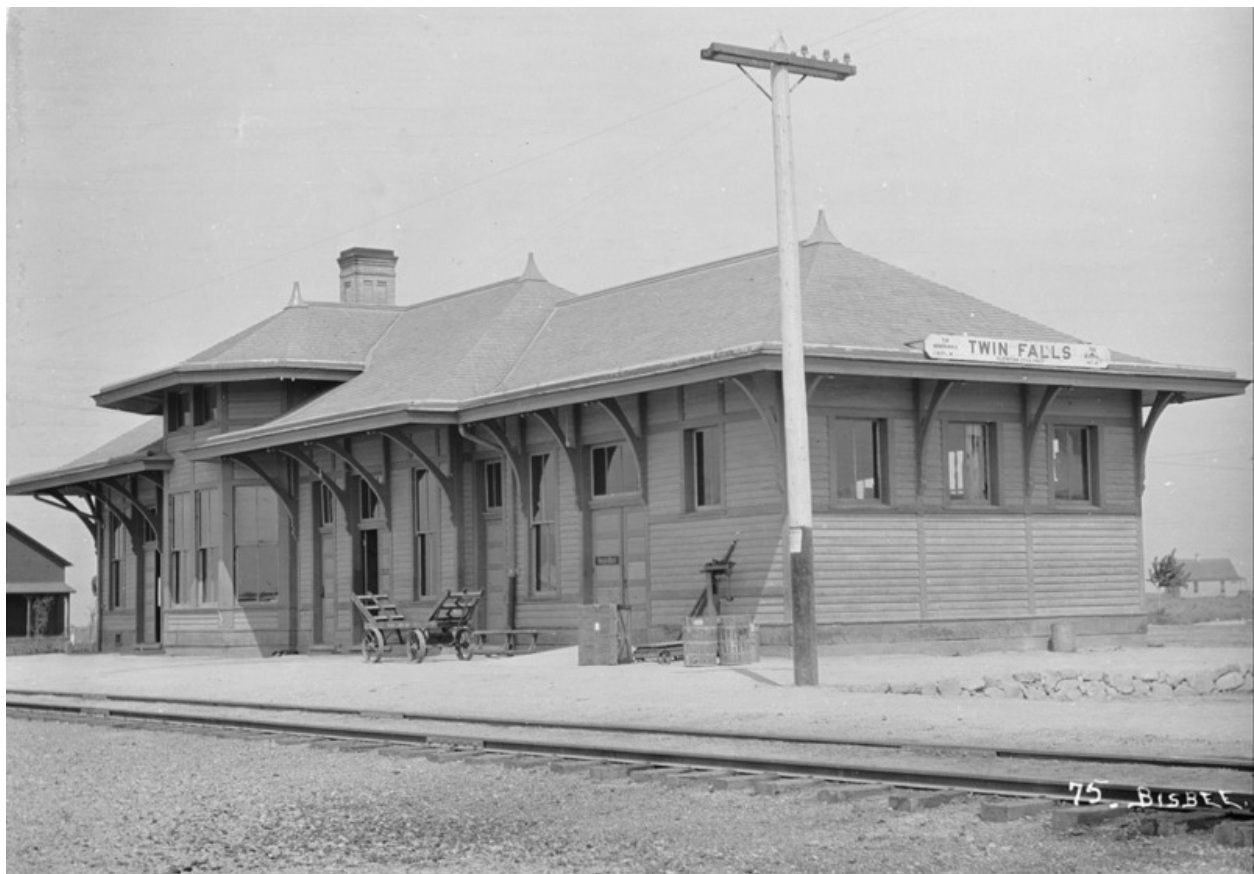
Building was across the street from the Depot Grill site
