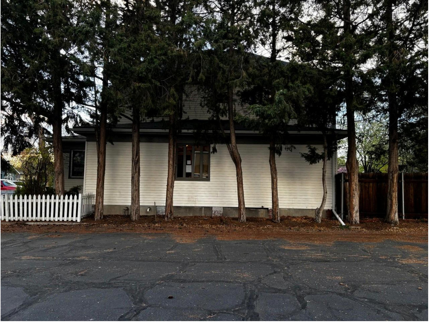
Existing Side Yard View
