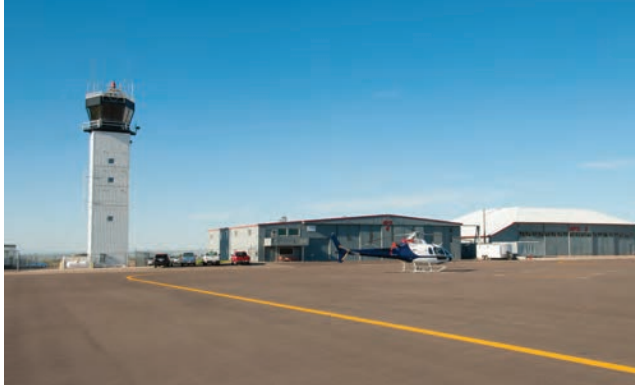
Tower and Apron
