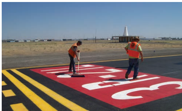
Taxiway D Rehabilitation
