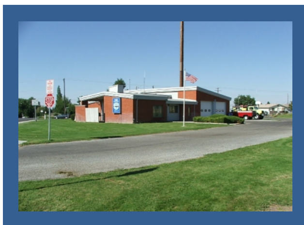
Figure 13: Twin Falls Fire Department Station 3
