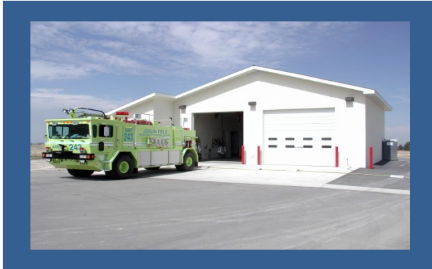
Figure 14: Twin Falls Fire Department Station 4
