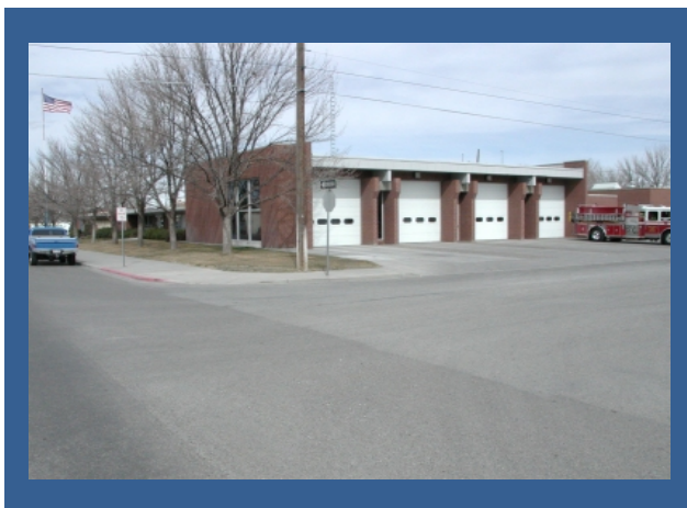
Figure 11: Twin Falls Fire Department Station 1
