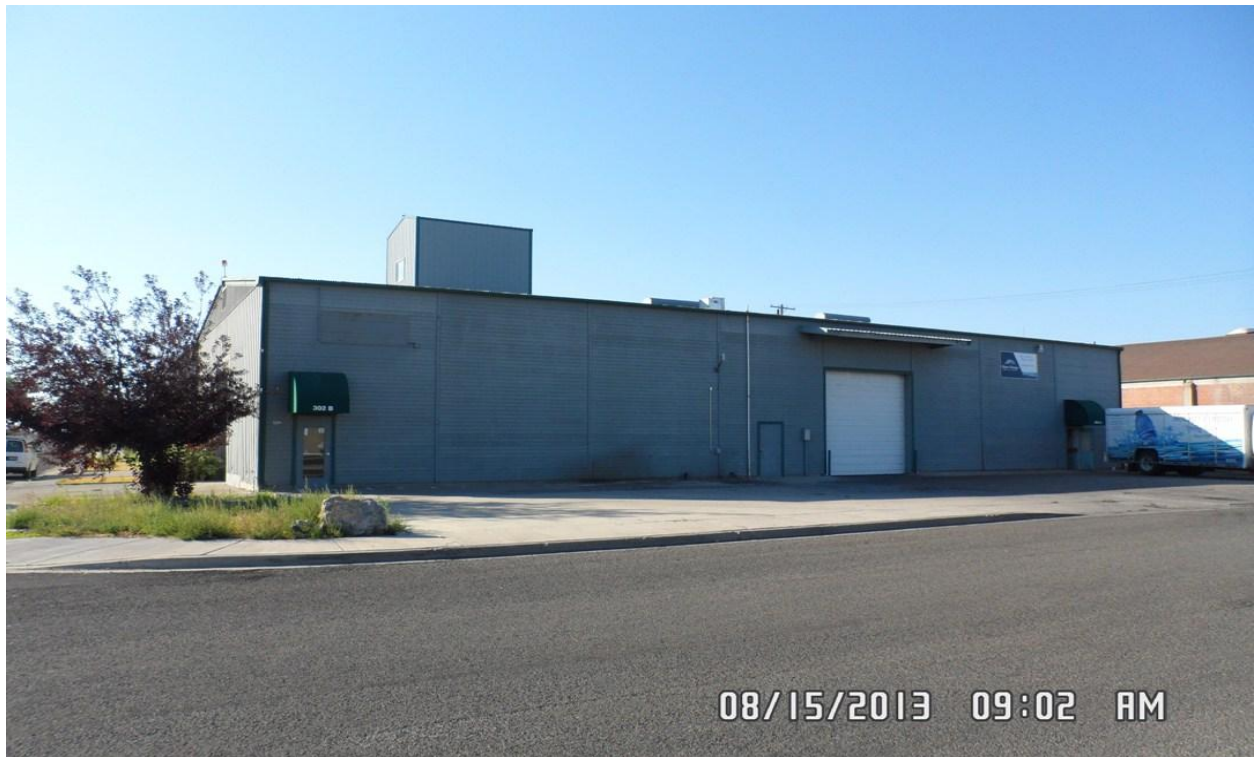
Northwest side of building.
