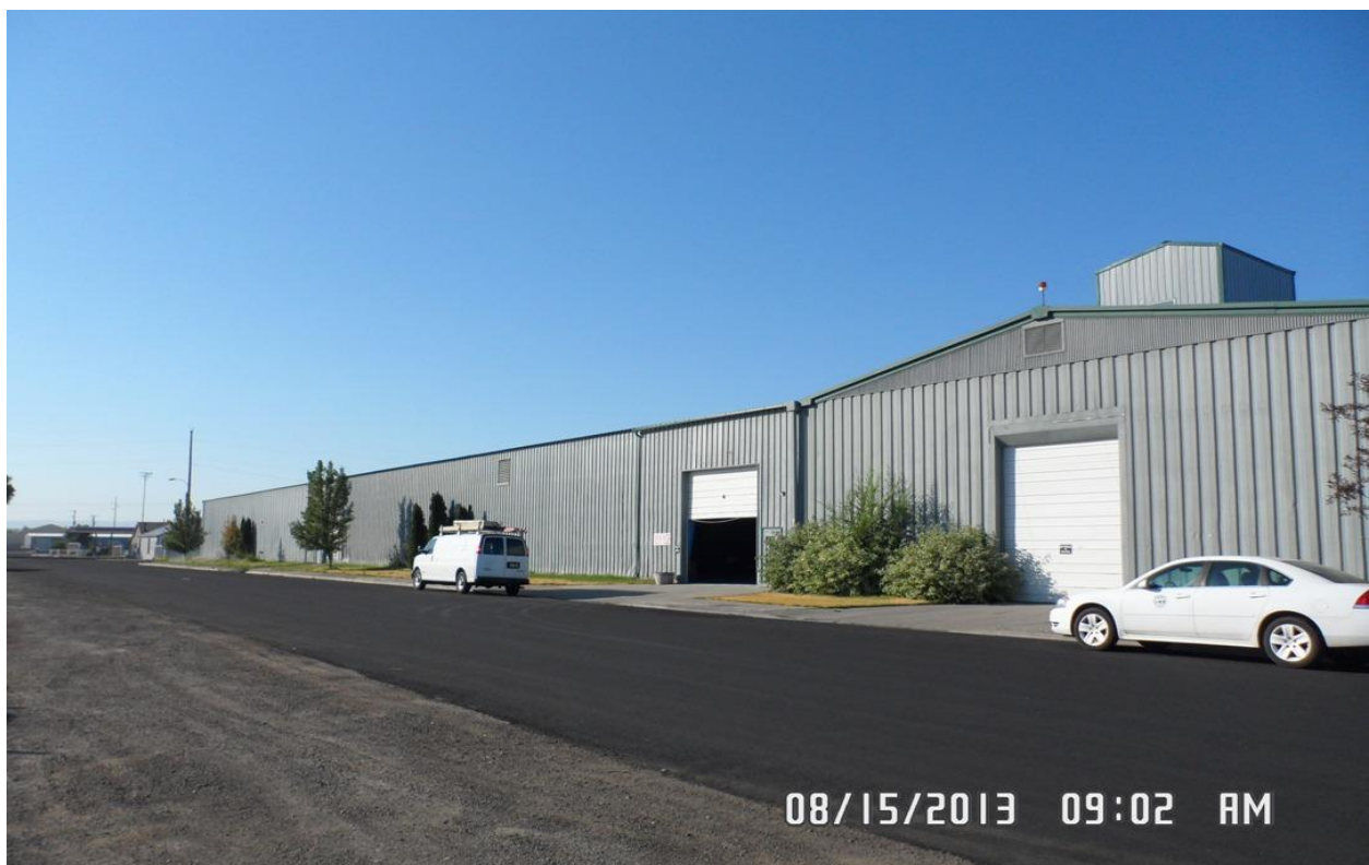
Northeast side of building.
