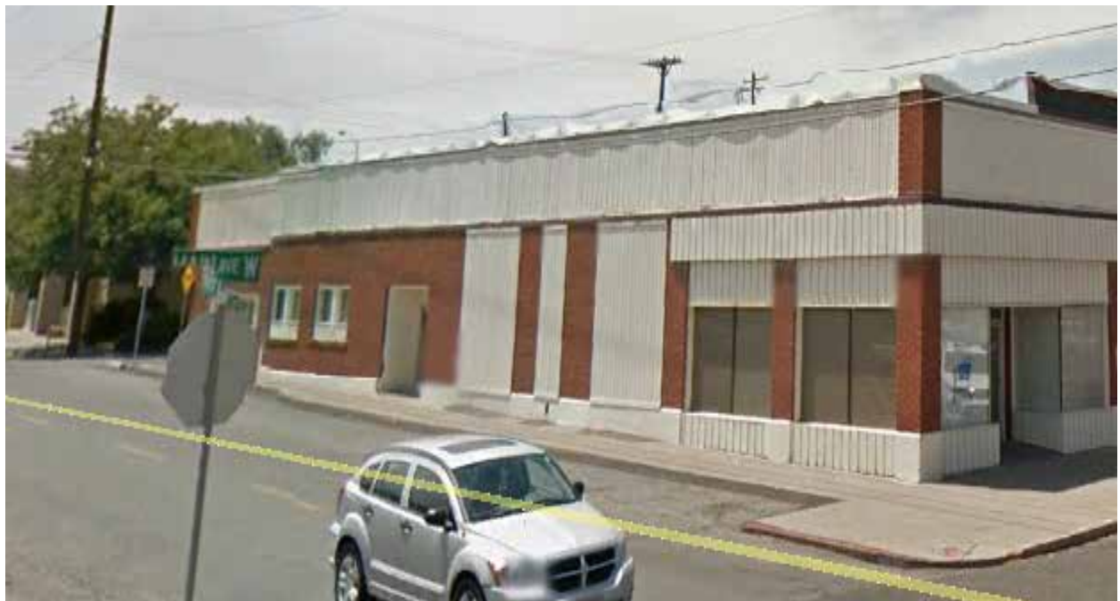
East side of building from Fairfield Ave W
