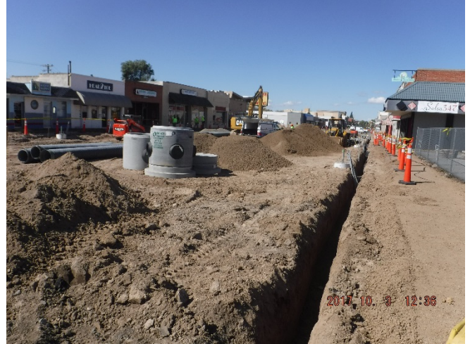
Block 5 – Idaho to Jerome, underground utility installation and preparing for sidewalk pour, 3OCT2017
