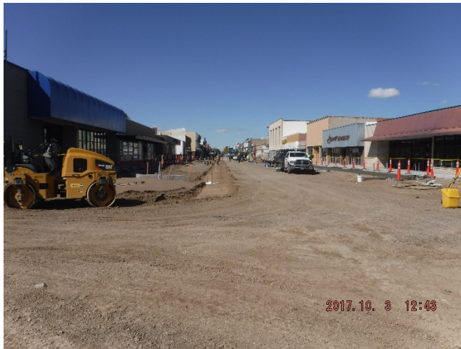
Block 4 – Hansen to Idaho, pouring curb and gutter, preparing for asphalt, 3OCT2017
