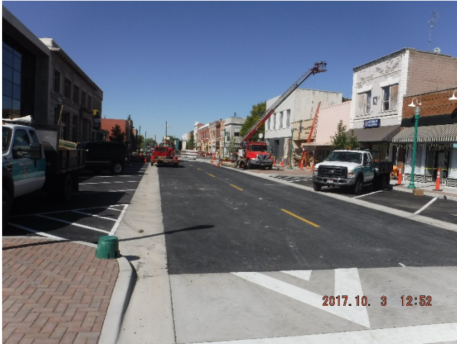
Block 3 – Shoshone to Hansen, Block nearly ready to be opened to traffic, 3OCT2017
