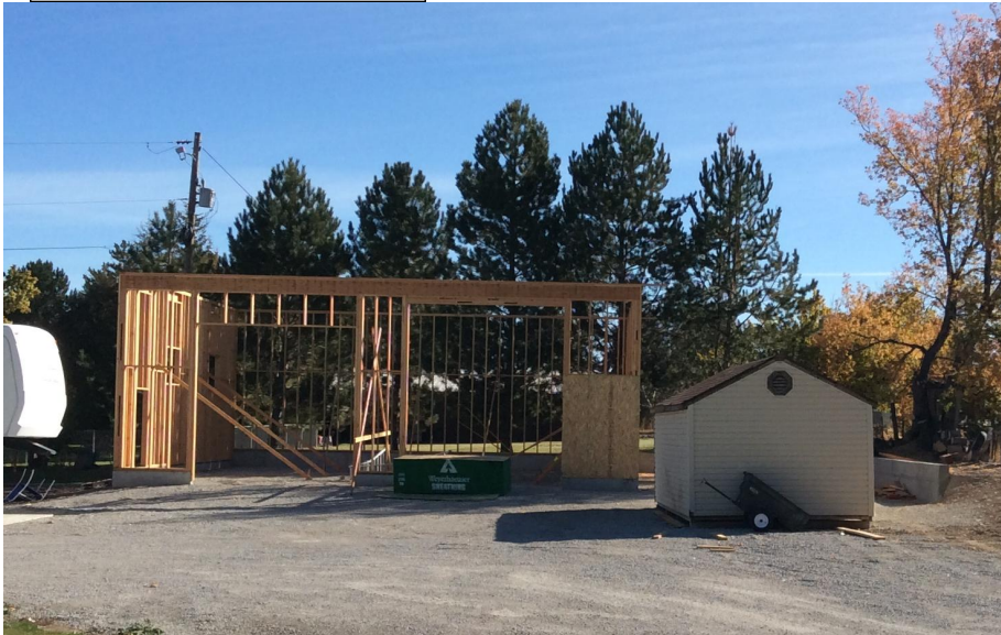
NW Corner Looking SE
