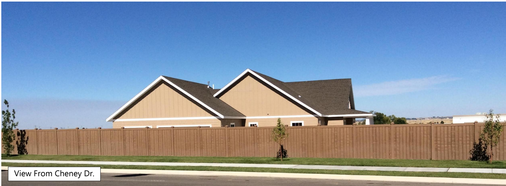
South Face of House
