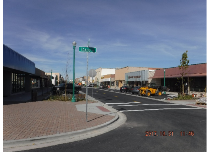
Block 4 –Hansen to Idaho, Block open to traffic, 31OCT2017
