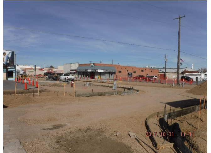
Block 5 – Idaho to Jerome, pouring curb and gutter, preparing for asphalt, 31OCT2017
