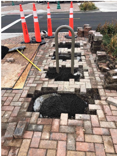
Bicycle Rack Installation, 27NOV2017
