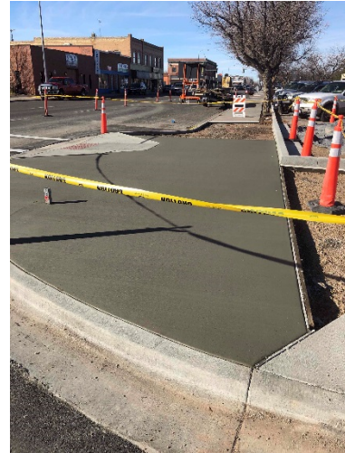
Block 6 – Hansen St S., Sidewalk pour, 28NOV2017
