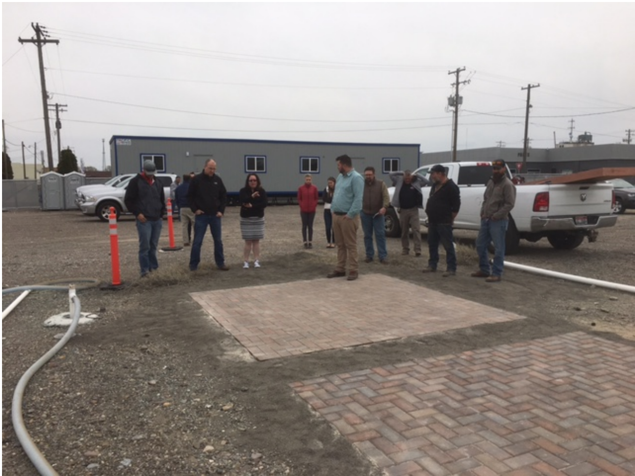
Brick Paver Mockup at Guho's Construction Yard, 11APR2017. The beveled "Holland Stone" pavers are in the section in the front of the photo (furthest from the group).
