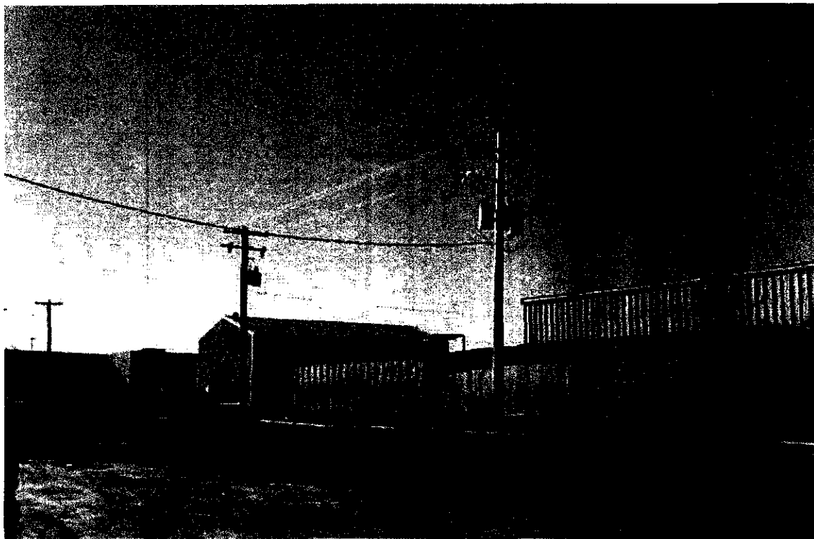
Photo 8: View of the western- southwestern adjoining properties with pole mounted transformers.
