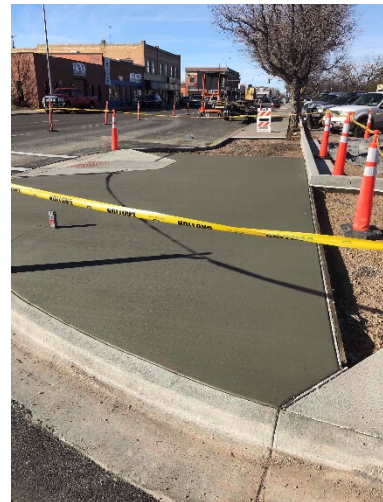
Block 6 – Hansen St S., Sidewalk pour, 28NOV2017
