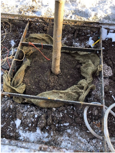
Replacement Tree Installation, 29DEC2017
