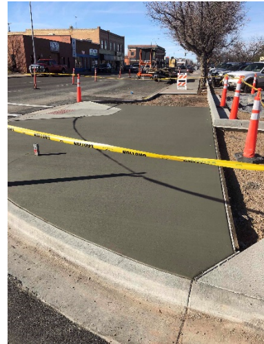
Block 6 – Hansen St S., Sidewalk pour, 28NOV2017
