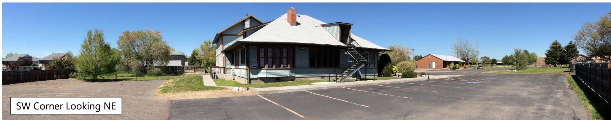
Rear of Building Looking East
