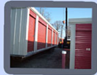
3 Crane Hooks Up
