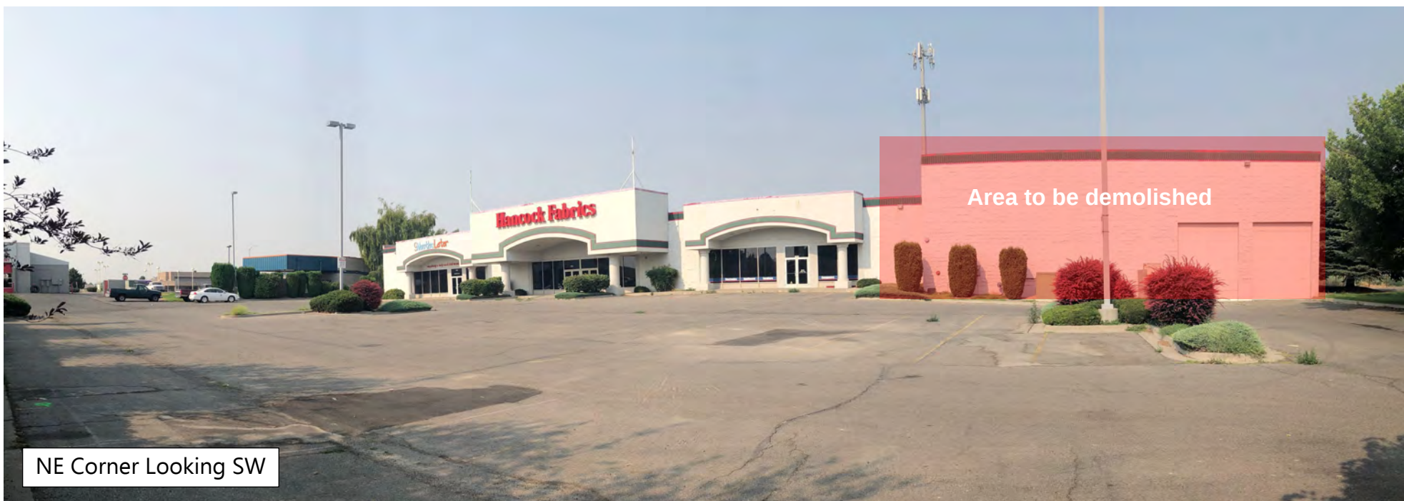
SE Corner Looking NW
