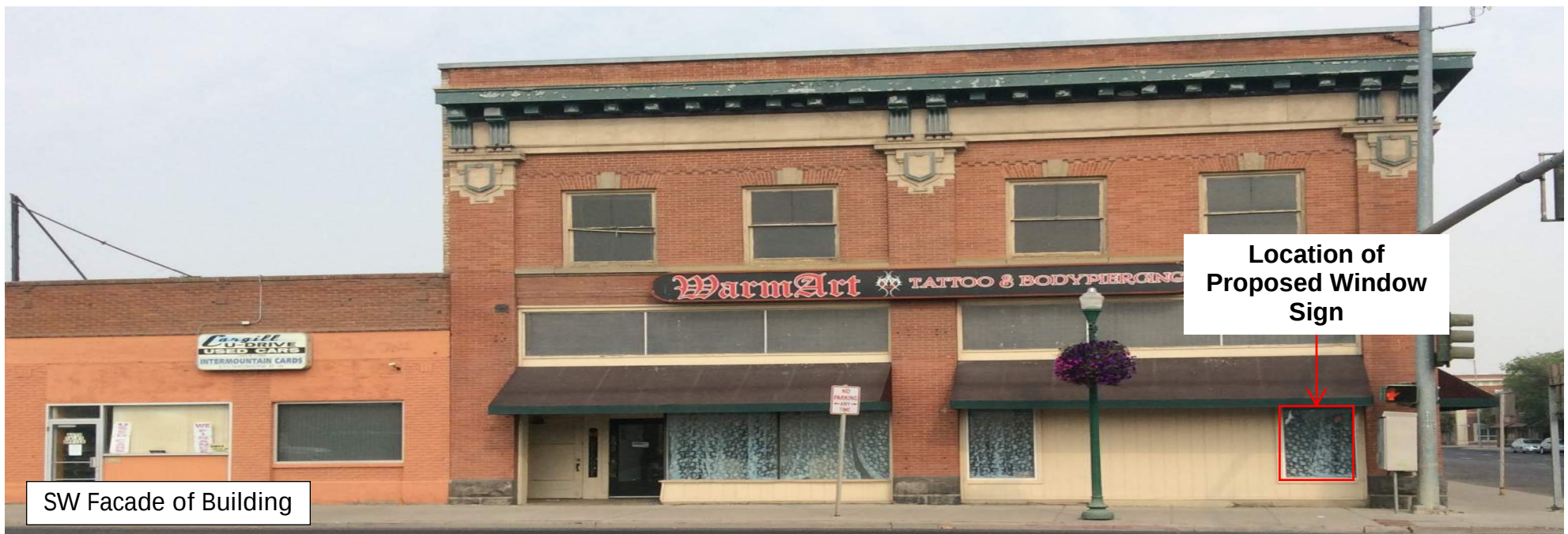
NE Facade of Building
