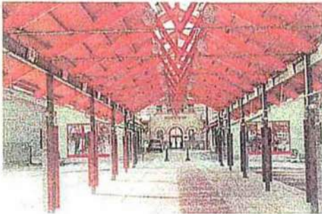
Farmers market permanent structure with parking in either side.
