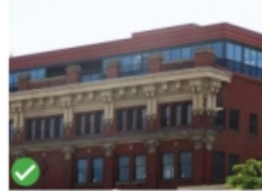
Appropriate setback of rooftop addition.
