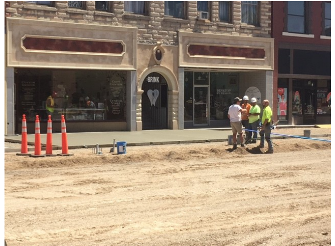
Concrete Sidewalk Placement on Main Ave. – Gooding to Shoshone; 06JUN2017
