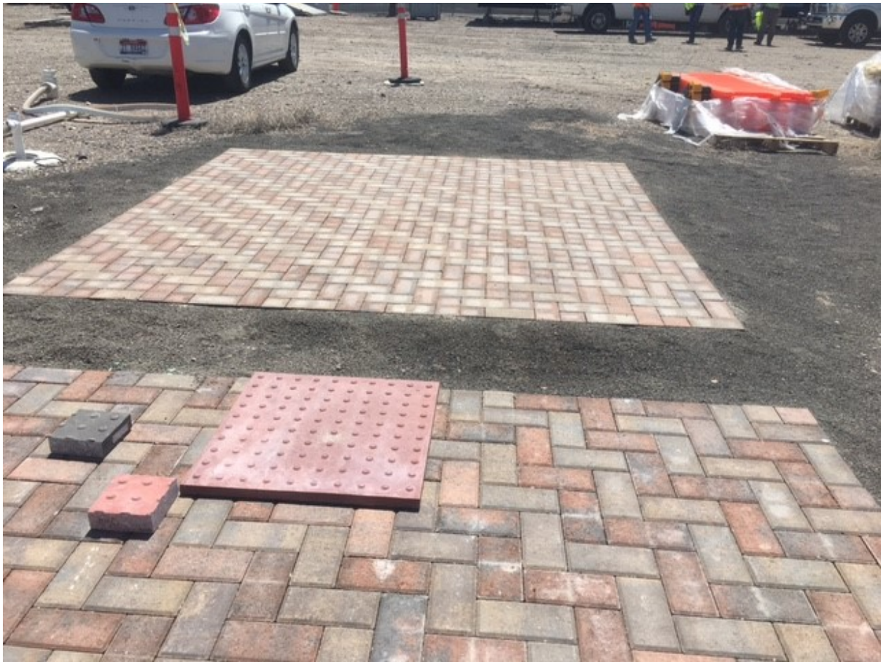
Truncated Dome selection for curb cuts, at paver mockup at Guho's construction yard, 06JUN2017. The beveled "Holland Stone" pavers are in the forefront of the photo, which have been selected for the Main Ave. Project.
