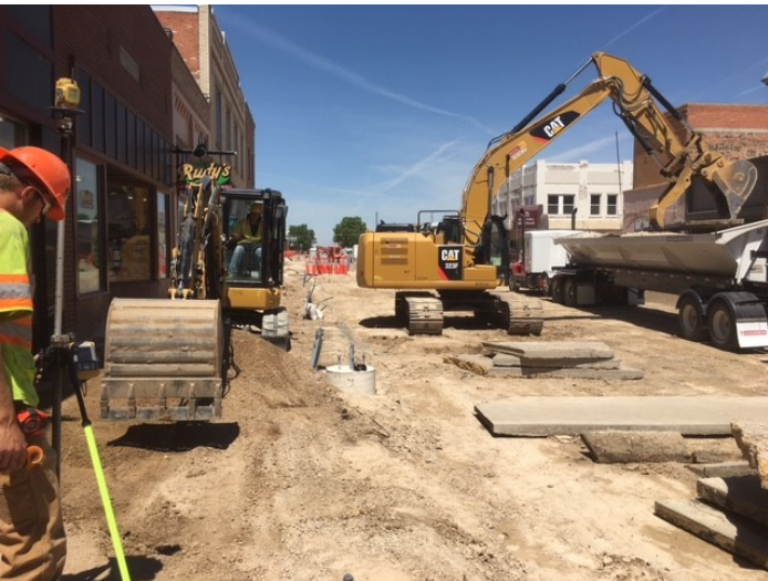
Existing Sidewalk Removal on Main Ave. - Gooding to Shoshone, 06JUN2017
