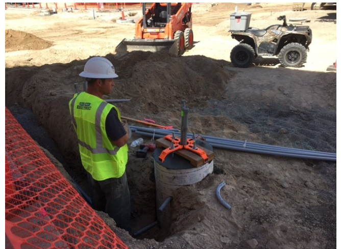
Light Pole Bases on main Ave. – Gooding to Shoshone, 02JUN2017
