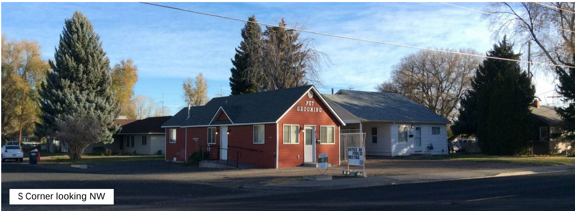
South Facade of Building
