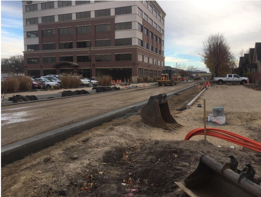
Similar Streetscape Project underway by Guho Corp in Boise, 22NOV2016
