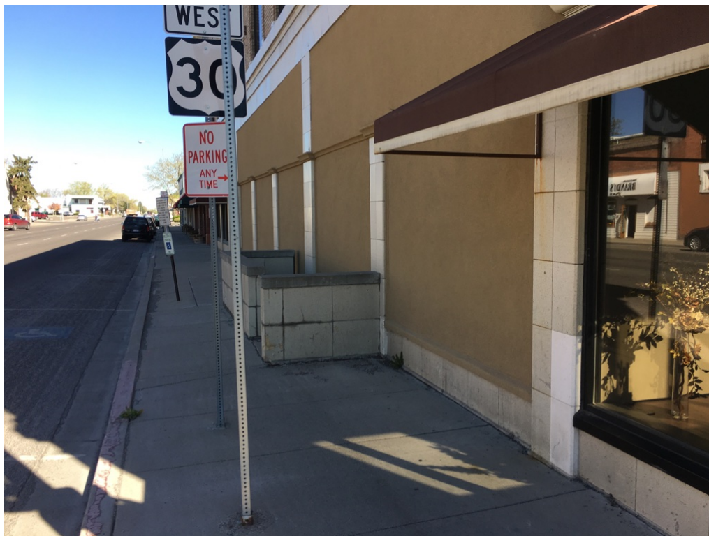
This photo shows again the 2 nd Avenue North façade which the applicant intends to restore.
