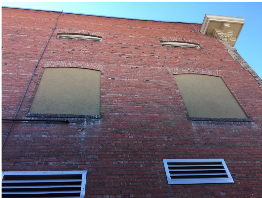
This photo shows the alleyway perpendicular to 2 nd Avenue North. The applicant intends to replace the large stucco cavities with windows.
