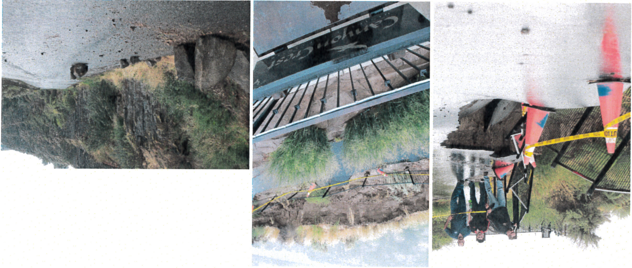
June 2006. Left photo: excavator removing loose rock following rockfall on Canyon Springs Road. Right photo: cleared rockfall on road and large fractures in tan rock above. Photo by Times News. Right photo: Photo by Shawn Willsey
