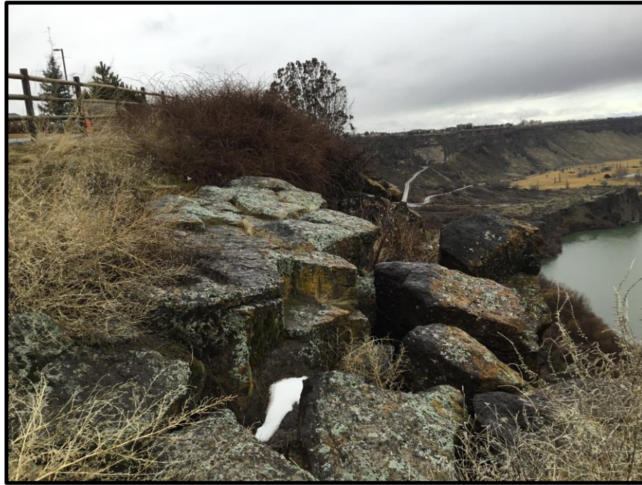
Photograph 3. Site conditions, looking west at the discontinuities in the basalt at the canyon rim north of the project site. Spacing of discontinuities is approximately 24 inches wide in photograph.
