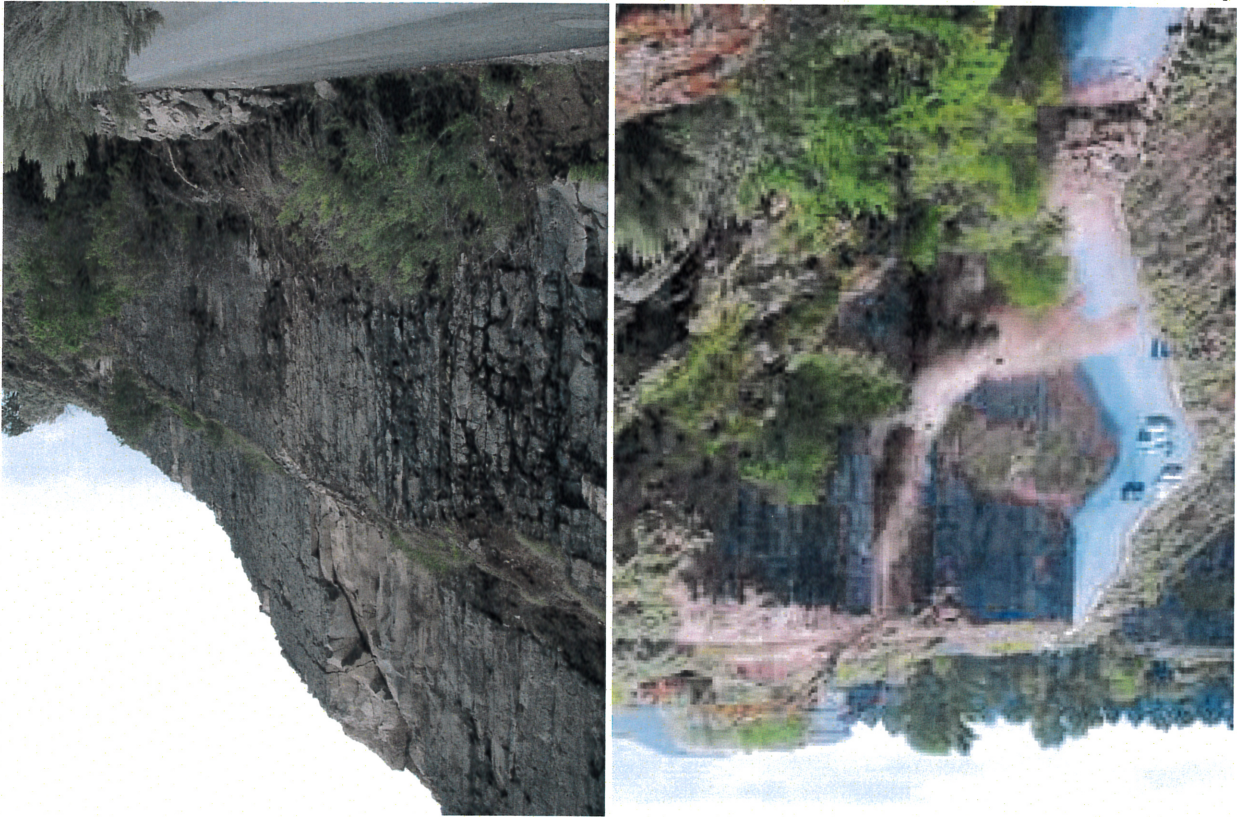
June 2006. Left photo: excavator removing loose rock following rockfall on Canyon Springs Road. Right photo: cleared rockfall on road and large fractures in tan rock above. Photo by Times News. Right photo: Photo by Shawn Willsey
