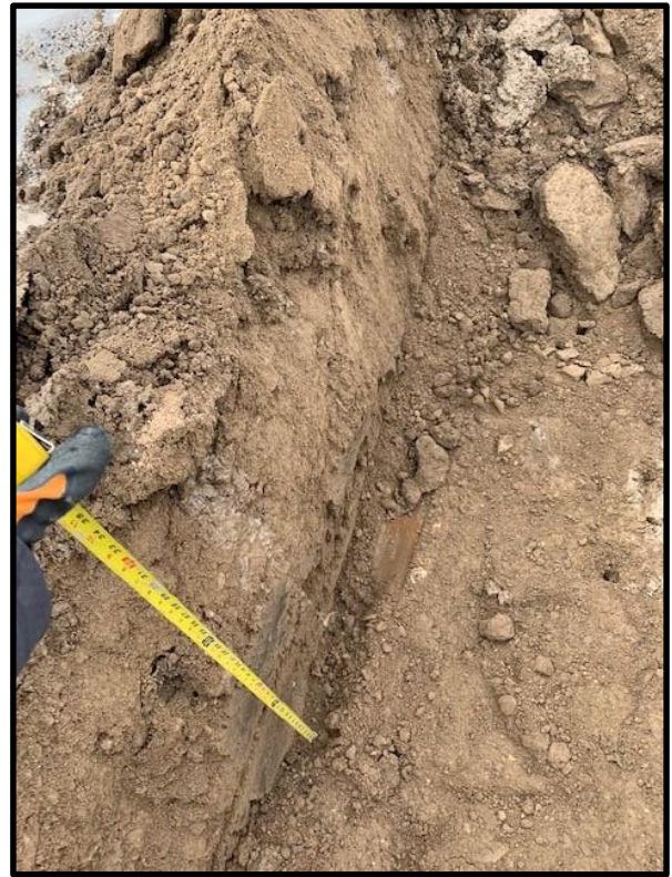
Photograph 14. Site conditions, excavation of TP-2.
