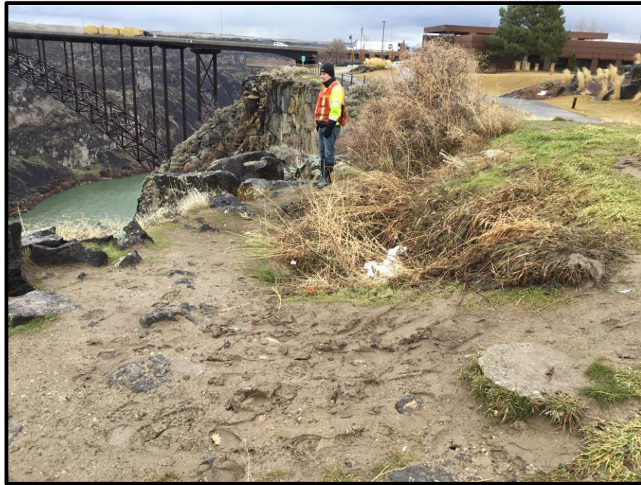
Photograph 7. Site conditions, looking south at canyon rim, north of the project site. Vegetation obscures tension cracks upslope of the canyon rim. Geologist in background represents the southern extent of the tension crack.
