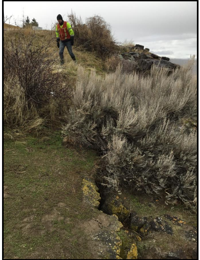
Photograph 6. Site conditions, looking at 2-inch wide discontinuity north of the project site. The geologist in the background of photo marks the northern extent of this discontinuity.
