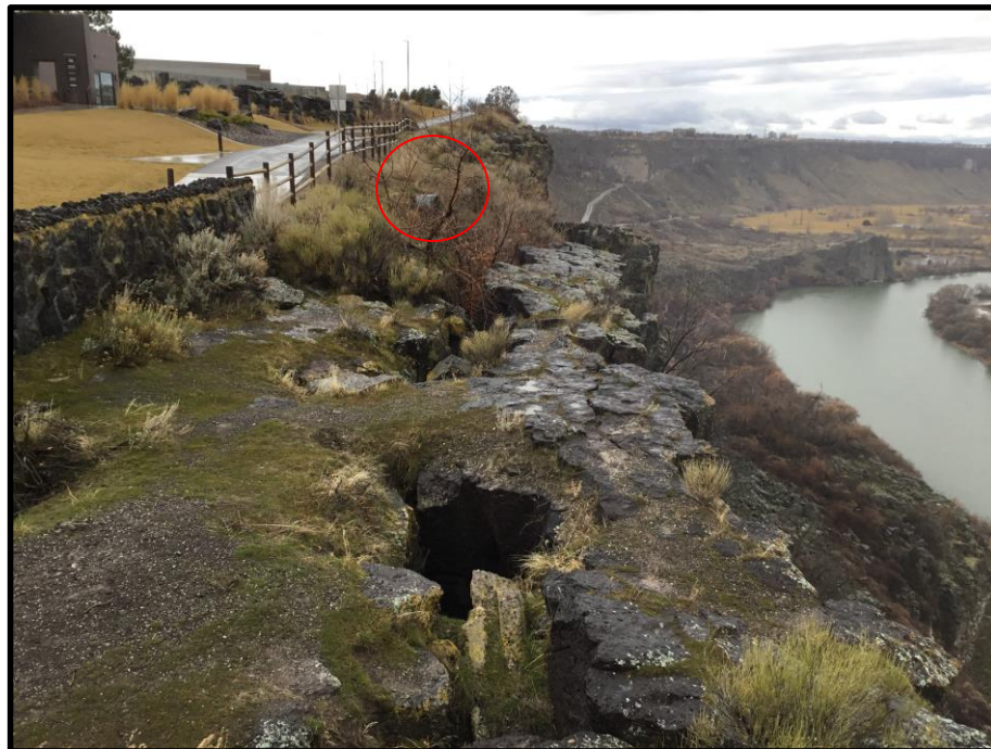
Photograph 8. Site conditions, looking west from Twin Falls Visitor Center Over look at drainage water runoff and 2-foot-wide tension crack. The red circle indicates outlet of drainage water runoff that was actively draining at time of geology reconnaissance.
