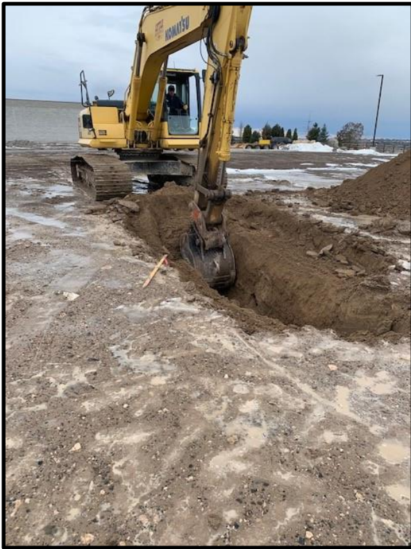
Photograph 13. Site conditions, excavation of TP-1.
