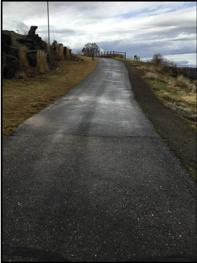
Photograph 9. Site conditions, looking north along paved walking path north of project site at pavement conditions. Pavement appears to be in good condition with no cracking observed.
