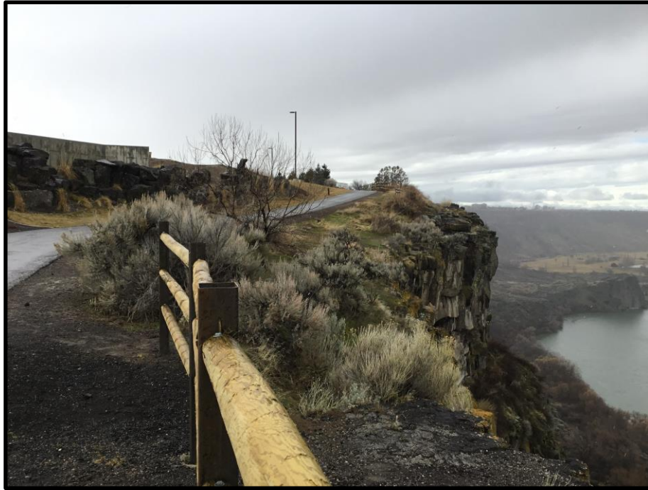
Photograph 1. Site condition, looking west from the northeast corner of the project site.
