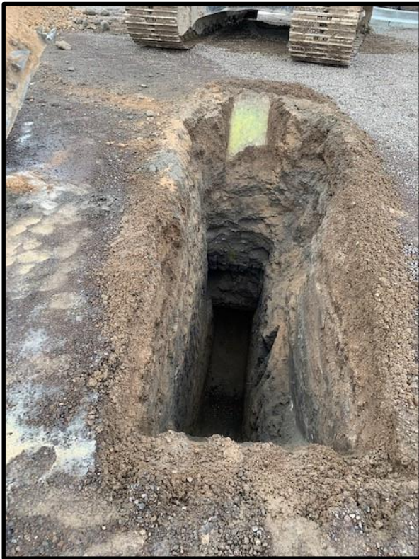
Photograph 15. Site conditions, excavation of TP-3.
