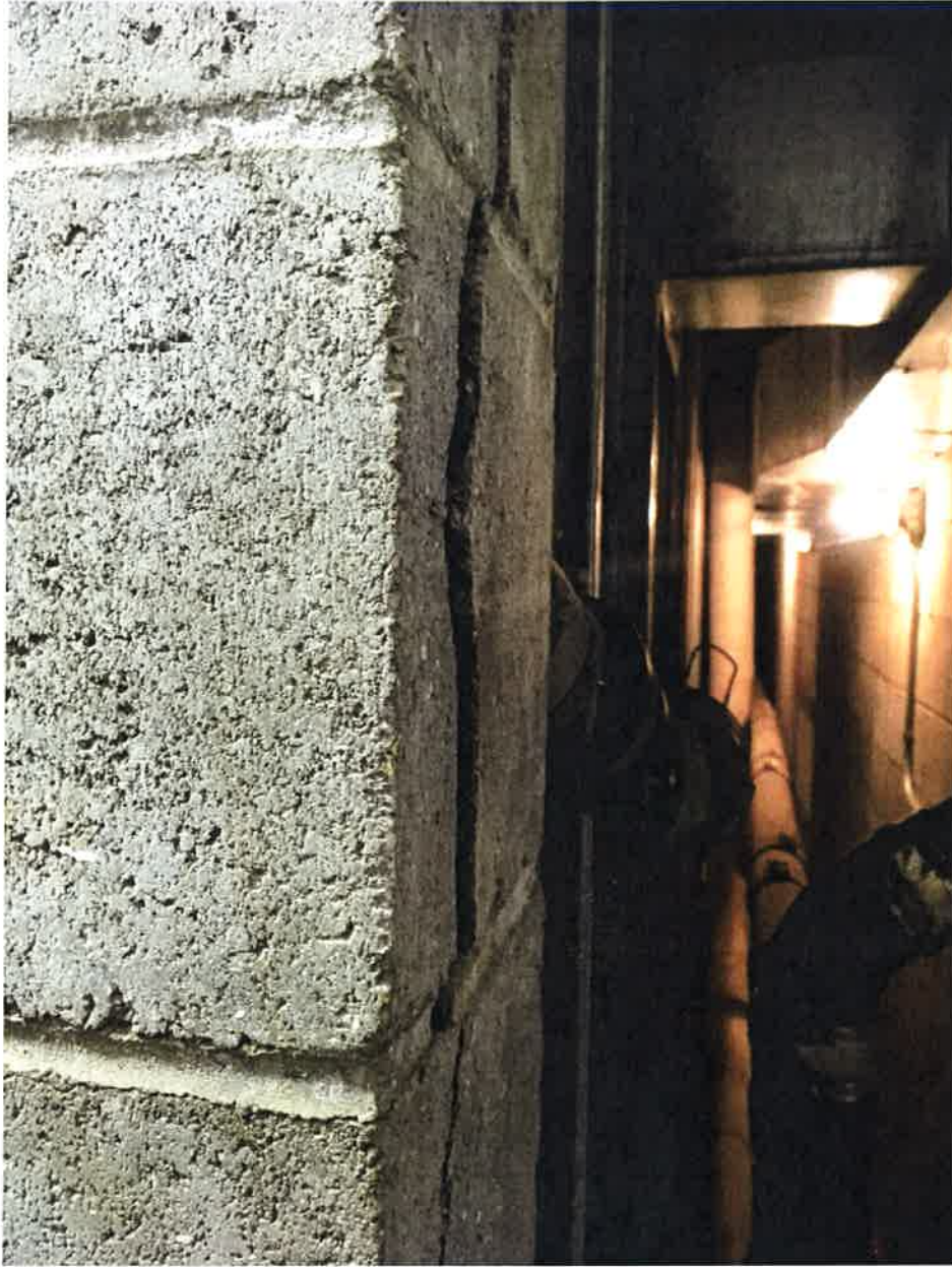
End of masonry wall below mezzanine floor. Looking north in plumbing chase.
