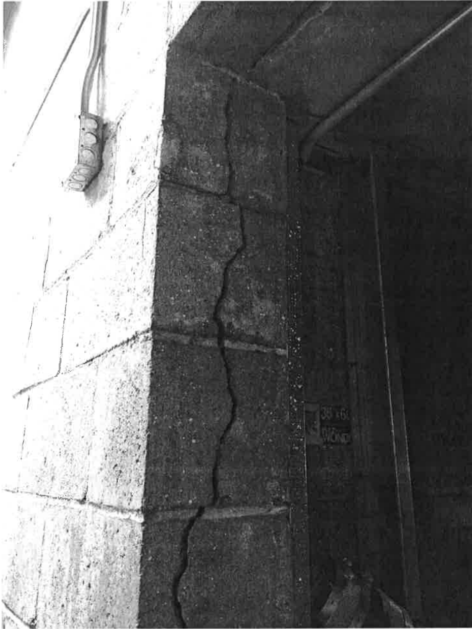
End of masonry wall below Mezzanine Floor
