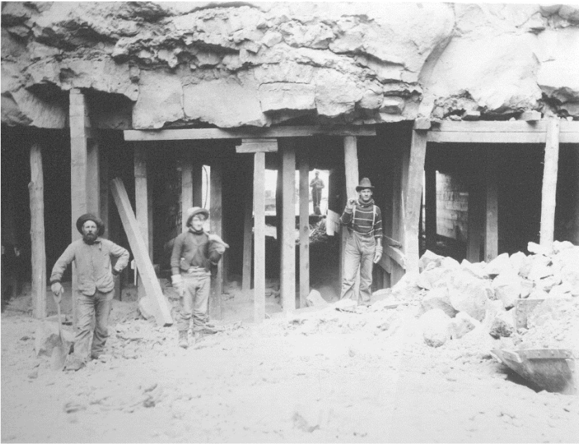
Picture Description: Without the dam-provided irrigation water, Twin Falls had no agriculture future. The construction of Milner Dam began in 1903, employing over 500 men. This image shows men with shovels at the mouth of the tunnel in 1904.
