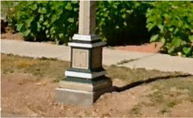
Figure 1. Light on 275 Lincoln Street. Homeowner reset the light that had been leaning. Base is not in original 6" border level and adjacent to curb.
