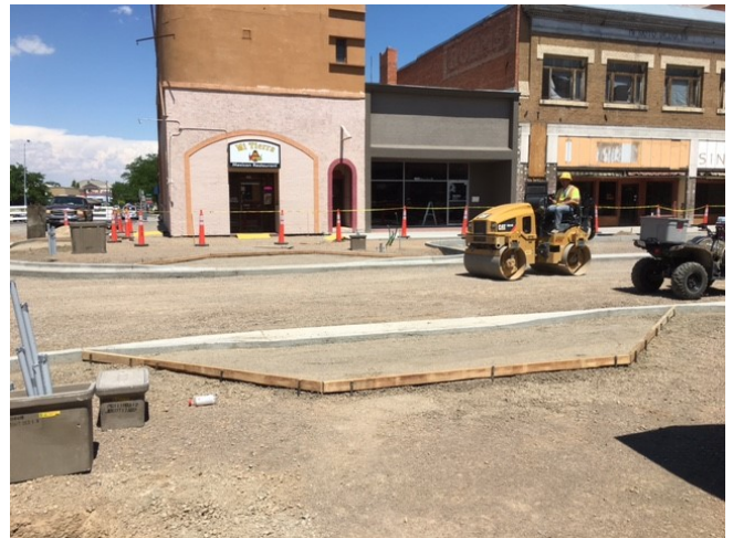
Block 2 – Fairfield to Gooding, prep for concrete and paver sidewalks, 28JUN2017
