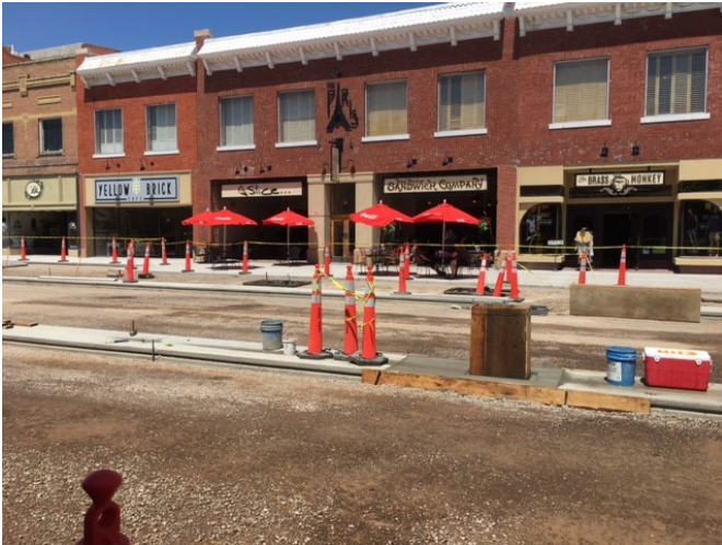
Block 1 – Shoshone to Gooding, concrete is placed with final prep for asphalt paving, 28JUN2017
