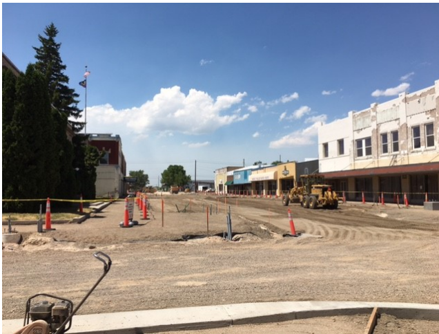
Block 2 – Fairfield to Gooding, storm drainage and power is complete; prep for concrete, 28JUN2017
