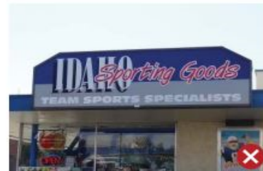
Inappropriate plastic, backlit sign.
