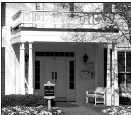
Smaller scaled signs on low posts are appropriate choices for offices in historic residential buildings.
