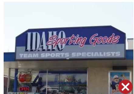
Inappropriate plastic, backlit sign.
