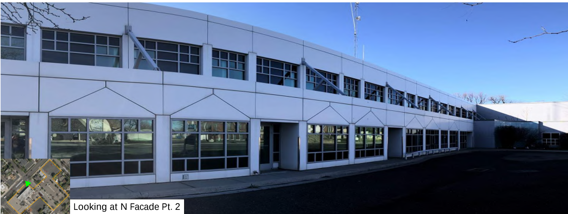
Looking at N Facade
